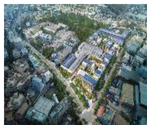
248-252 Pireos str. – Reconstruction of former industrial building Athens
