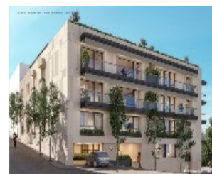
40-42 Ardittou str., Mets – Reconstruction of building Athens
