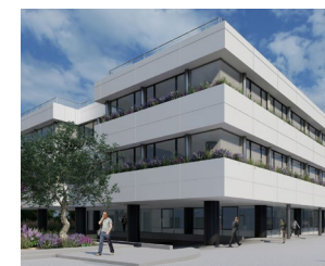
16 Chimarras str., Marousi – Construction of new office building Athens
