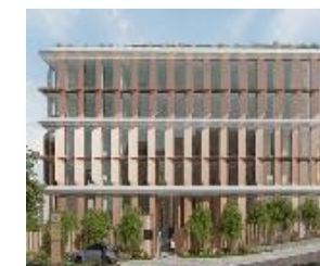
199 Kifisias Ave. Marousi – Reconstruction of existing office building Athens
